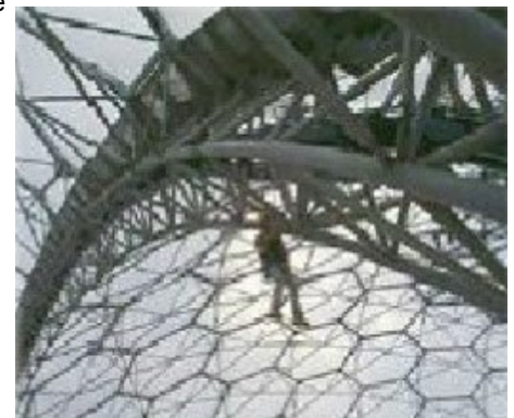
Lizard® inspection of geodetic structure using rope access operators
