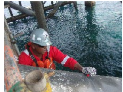
Offshore rope access inspections performed using the Lizard® M8 NDE System
