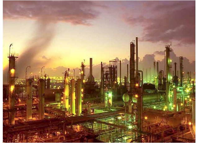
Hydro cracking plant where the principle application is the many internal trays and their attachment to the vessel walls with site welds and remedial grinding
