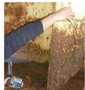
Port dock thickness measurement
