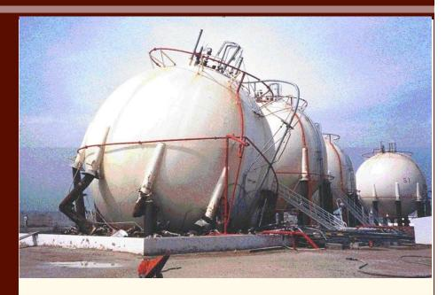
Don't let corrosion under fireproofing (CUF) weaken the legs holding up your gas storage spheres: Inspect for CUF using either the standard Bracelet Probe, pictured below, of the large Bracelet Probe used with our patented robotic crawler.
